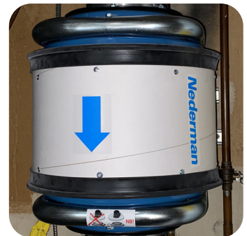
Nederman FX 2 HEPA filter is installed away from the patient area in the mechanical room.
